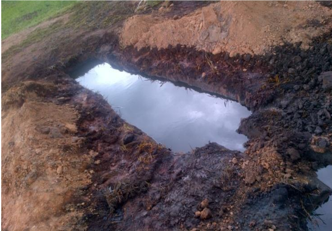
Spill point filled with oil on arrival
